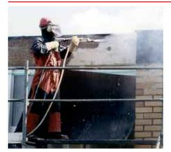
OERTZEN TORNADO - a wide range whirl sandblaster with high surface cleaning power and soft surface treatment.
