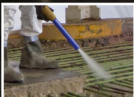
Concrete Repair and Restoration
